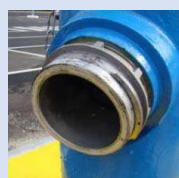
Raccord tournant
